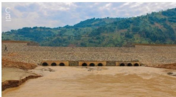
Figure 15&16: Muhazi dyke & Sebeya retention dam
