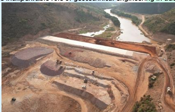
Figure 14: Construction of 80MW Rusumo Hydropower Dam
