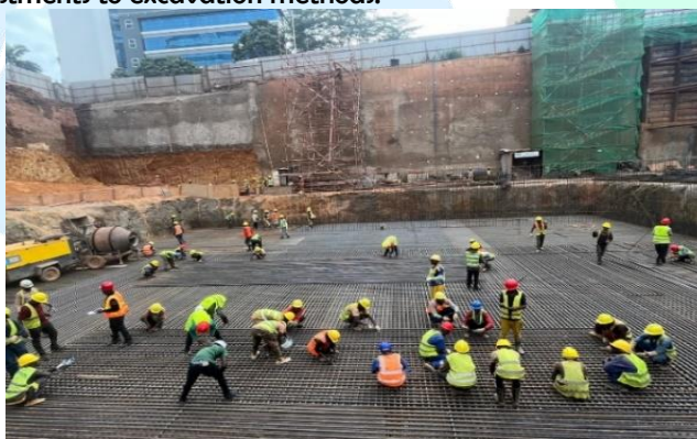
Figure 10: Deep excavation at Twin Tower Buildings at Kigali Financial Business Square
